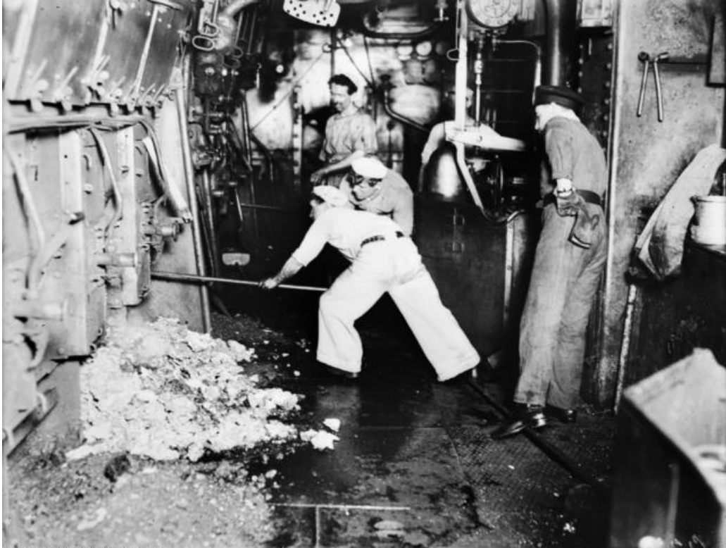
An unidentified stoker scrapes out the ash from the bottom grate in the boiler furnace on HMAS Australia . (Photo c 1918)
